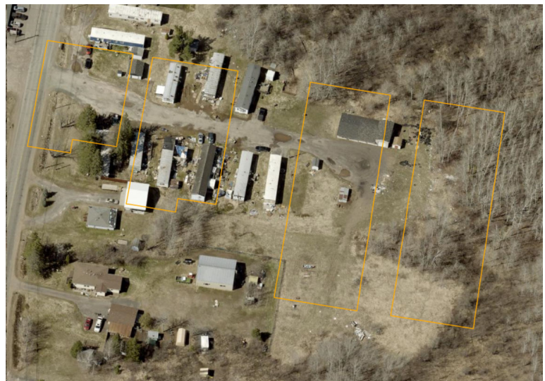
OBLIQUE AERIAL PHOTO VIEW FROM THE SOUTH
