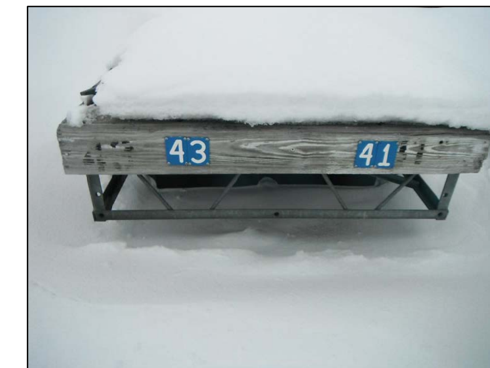
TYPICAL SLIP NUMBER LOCATION ON FINGER PIERS
