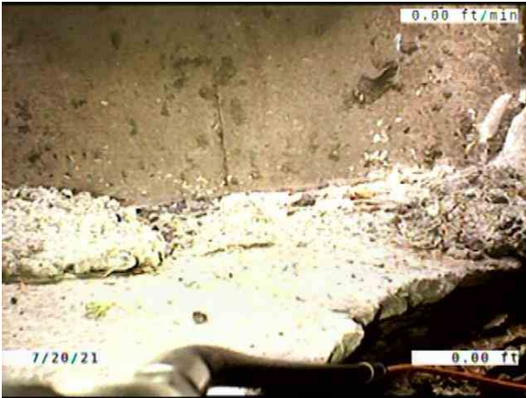
CB010016-CB01016A_4986dda5-b245-4260-84ef-57f3ec271a33_20210720_174858_647.jpg, 00:00:01, 0.00ft Catch Basin / CB010016
