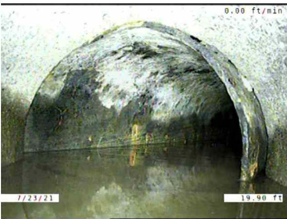
CB010025-CB01065B_932083d0-5c72-4a21-a2c2-394ed3a39dfb_20210723_130918_336.jpg, 00:08:19, 19.90ft Miscellaneous Survey Abandoned / CAMERA CANT MAKE IT PAST THE ANGLED JOINT
