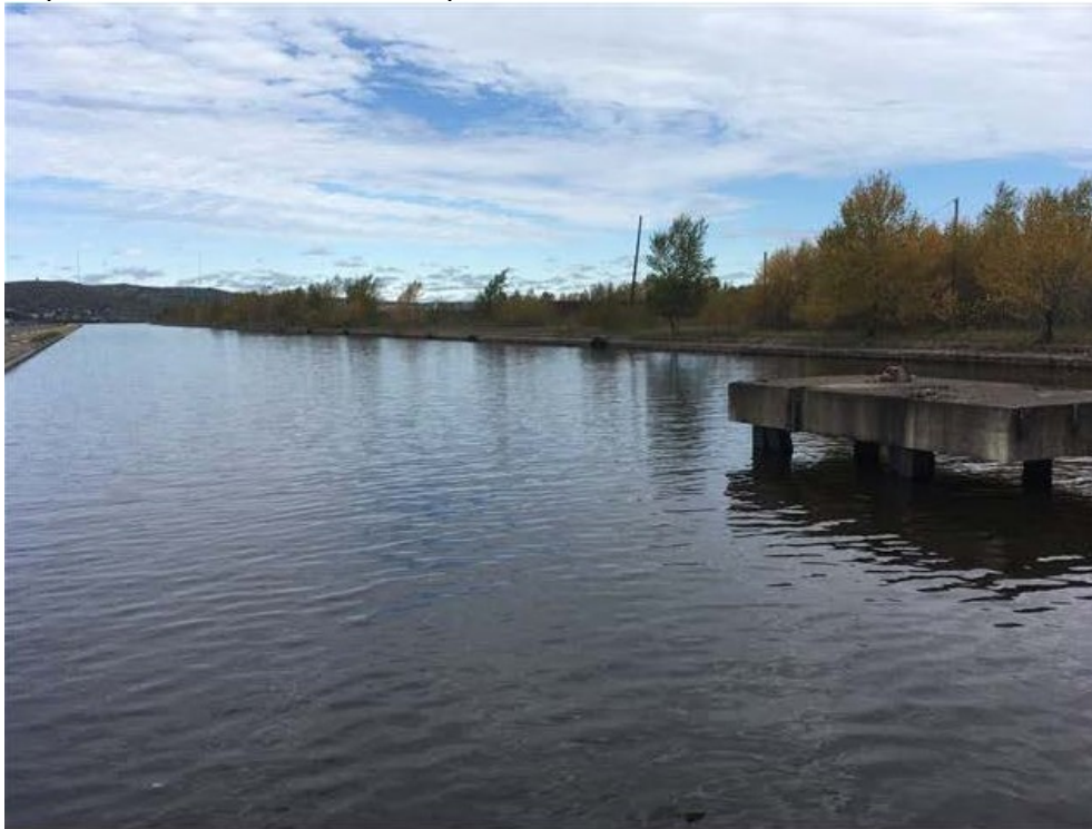
Dock wall and slip dredge area, approx. view looking northeast.
