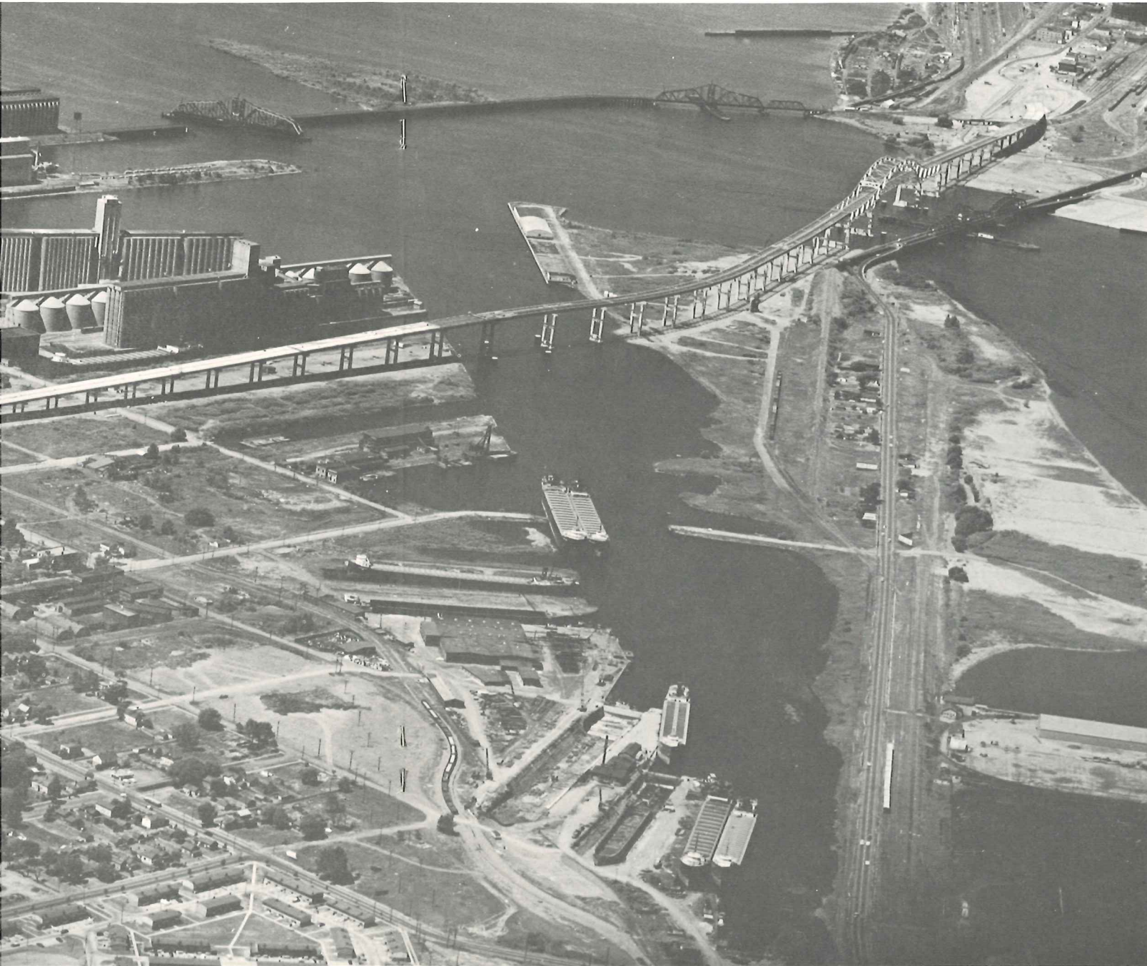
SH BRIDGE - LINKING SUPERIOR AND DULUTH - SUPERIOR-DULUTH HARBOR VIEW
