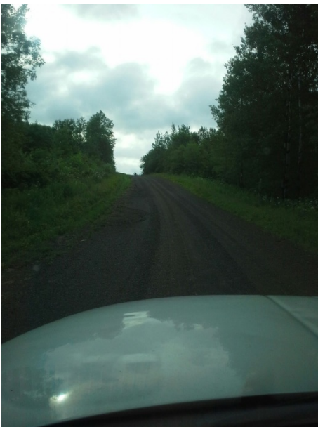
#4 Bardon Creek Rd hillside looking east
