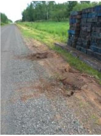
Camp Amn Rd Pipeline 1
