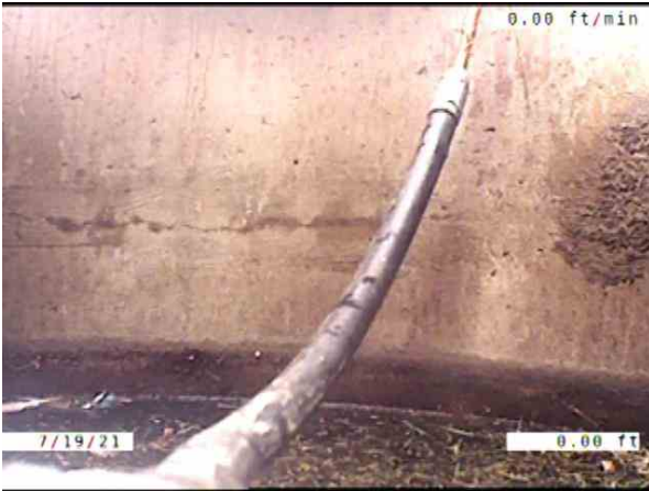
CB010024-CB010360_a333811d-b985-4dd3-b822-49f9d0d35226_20210719_155755_706.jpg, 00:00:01, 0.00ft Catch Basin / CB010024
