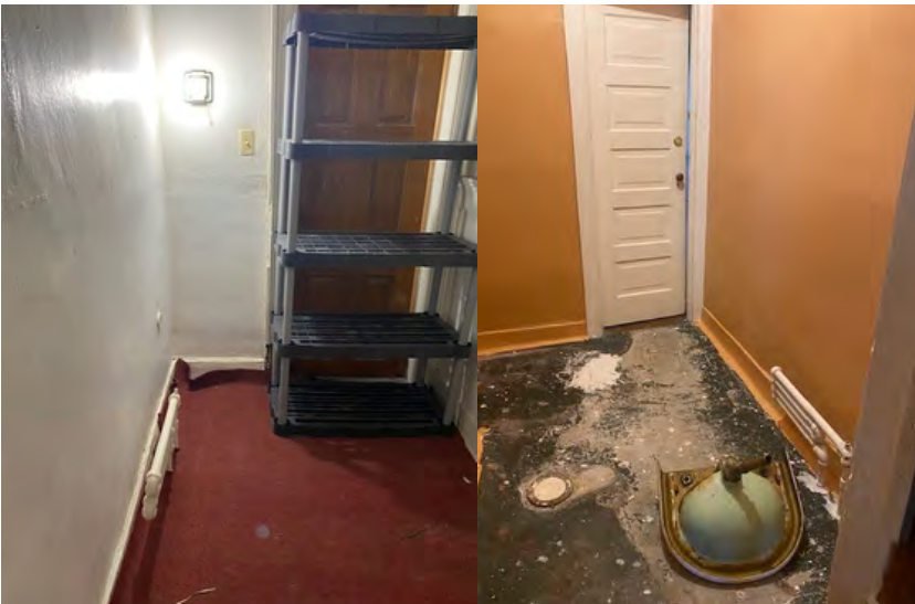
3rd floor bathroom at Fairlawn
