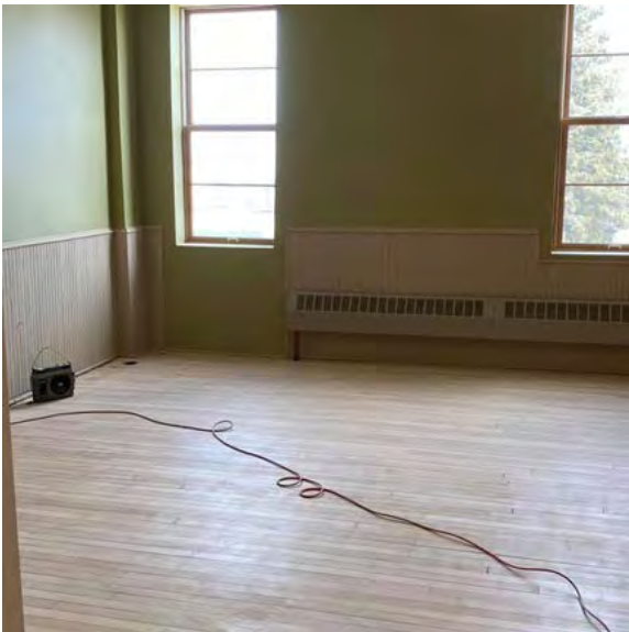
Completion of the Captain's Bedroom at the Old Firehouse & Police Museum.
