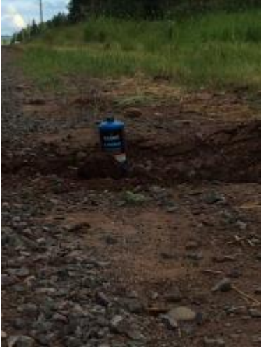
Camp Amn Rd Pipeline 2
