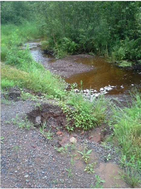
#1 Wouri Rd intersection with Lindgren Rd Looking south
