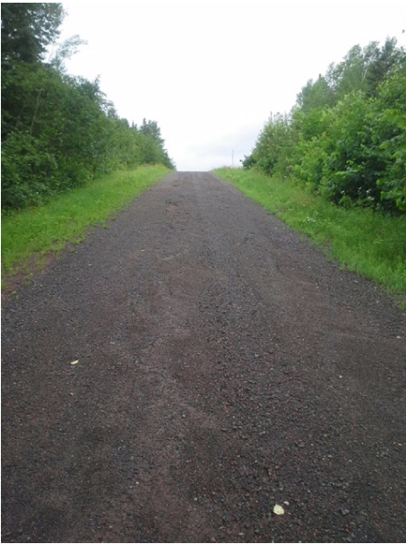
#5 Lund Rd hillside looking west
