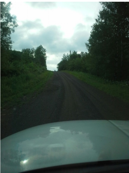
#4 Bardon Creek Rd hillside looking east
