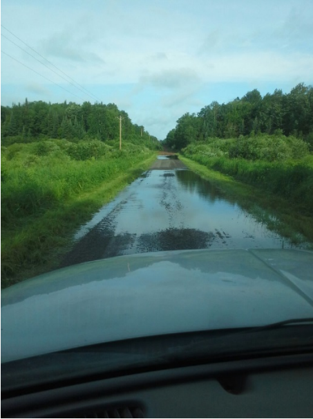
#3a East end of Blueberry Rd looking west
